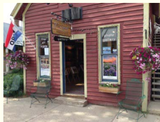
Store Front Windows
